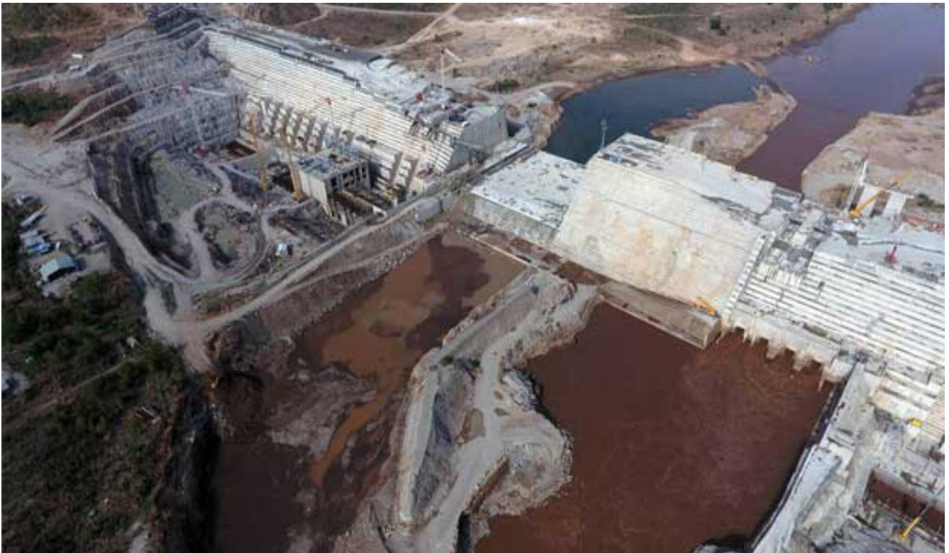
The Grand Ethiopian Renaissance Dam under construction in 2017 (courtesy of Salini Impregilo)
